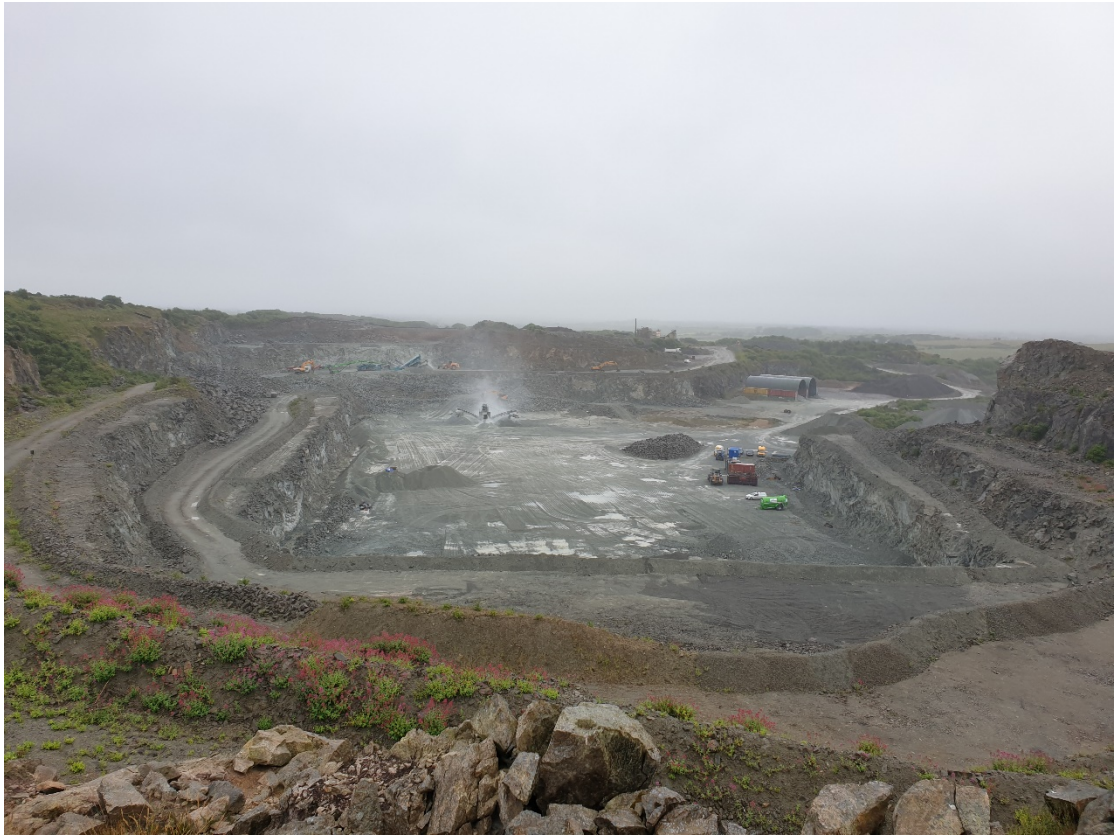
Plate 1: Shot of existing quarry to south of proposed extension area, looking south
